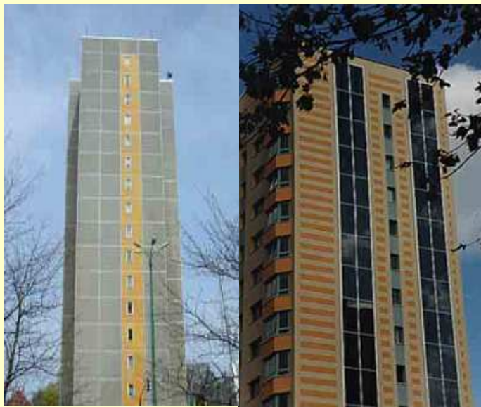
Renovation prefabricated apartment block- Potsdam, Germany – 2000
